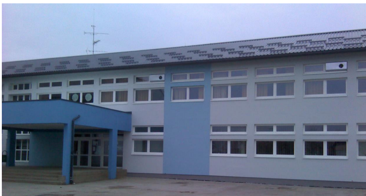
Figure 1 Reconstructed Primary school in Koprivnica
