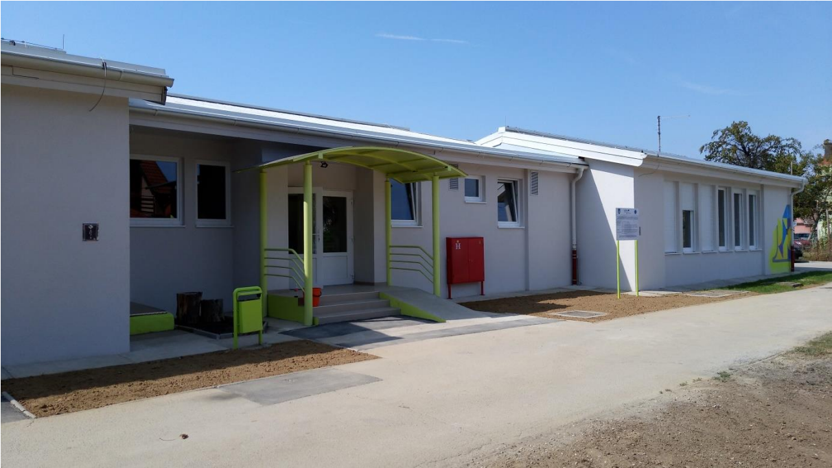
Figure 1 Reconstructed Kindergarten Loptica
