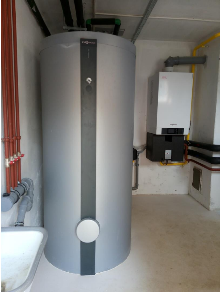
Figure 2 Reconstructed boiler room in Kindergarten Loptica
