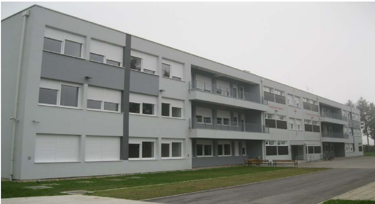
Figure 2 Reconstructed building in in former military complex
